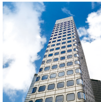
St. John's Building Hong Kong (office) Established: 1983 GFA: 71,400 sq. ft. Ownership: 100%
