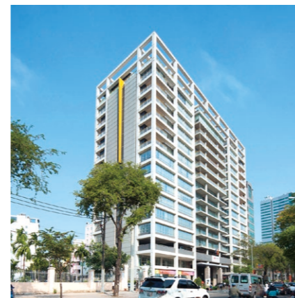
The Landmark Ho Chi Minh City, Vietnam (office and residential) Established: 1994 GFA: 175,903 sq. ft. Ownership: 70%
