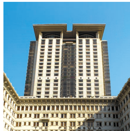
The Peninsula Office Tower Hong Kong Established: 1994 GFA: 75,082 sq. ft. Ownership: 100%
