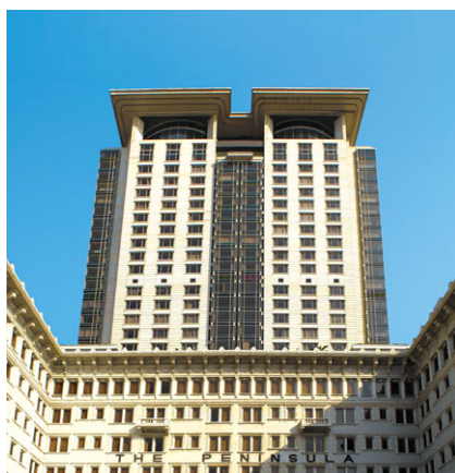
The Peninsula Office Tower Hong Kong Established: 1994 GFA: 75,082 sq. ft. Ownership: 100%
